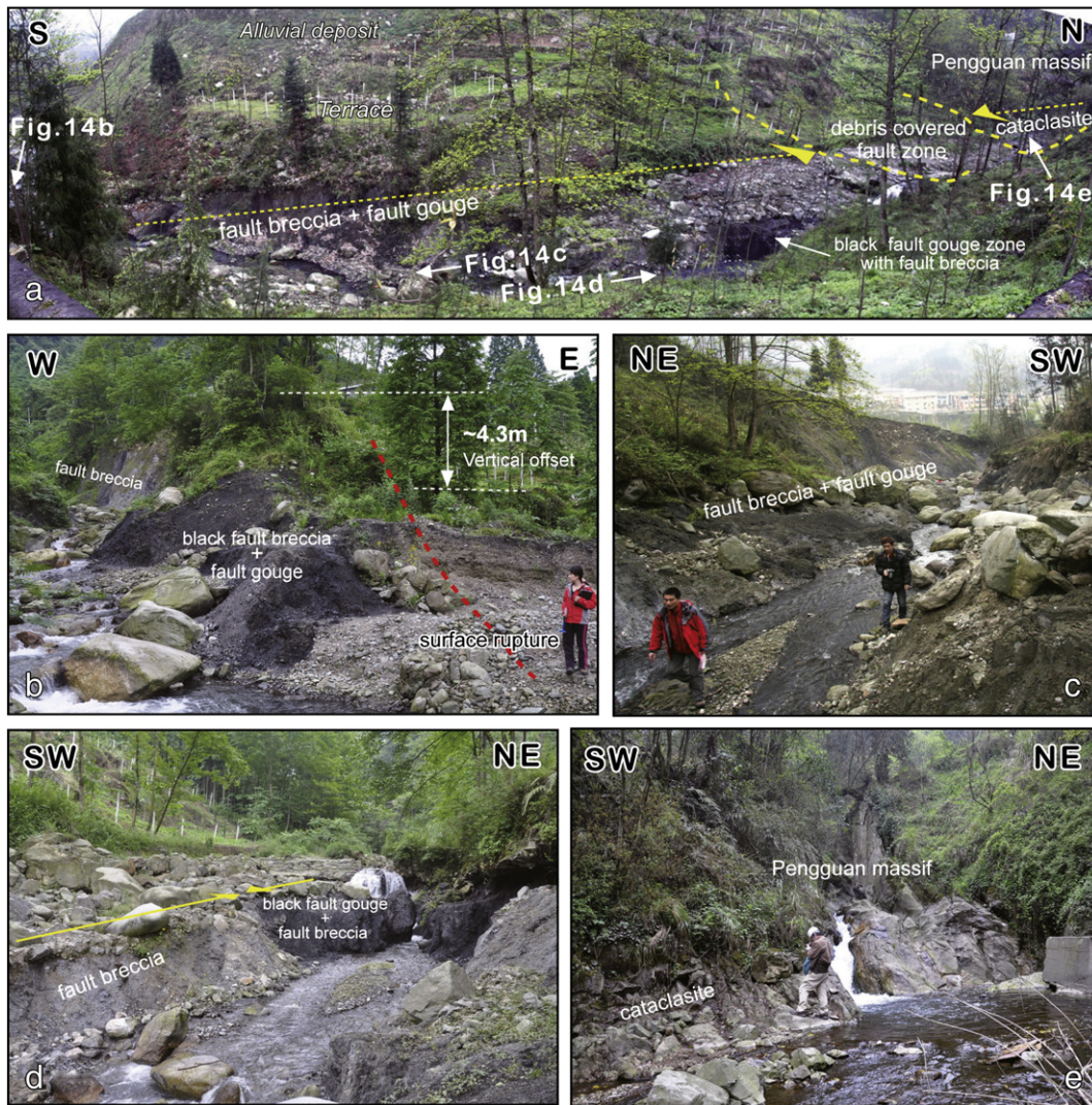
Fig. 14. Photos of outcrops of Yingxiu–Beichuan fault zone at Bajiaomiao village taken in March 2012. Location shown in Fig. 2. (a) Panoramic photo of the fault zone. Black fault zones (black fault gouges and/or black fault breccias) distribution at the bottom (b) and top (a, d) of the Xujiuhe formation. Gray fault breccia and fault gouge zone (c) distribution between them, and (e) Pengguan massif (the cataclasite zone) in the northern outcrop. The red dashed line represents the co-seismic surface rupture zone of the Wenchuan earthquake (b).
