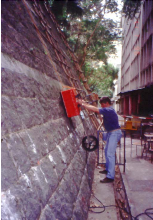
Geophysical surveys of slope and retaining wall
