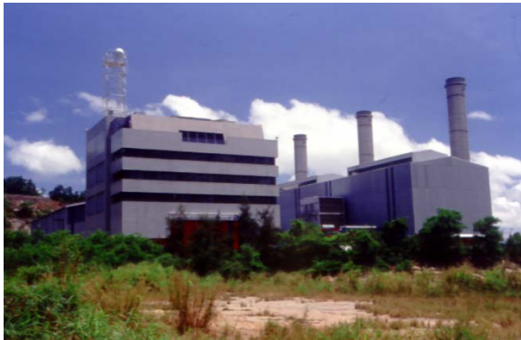
Penny's Bay Power Station
